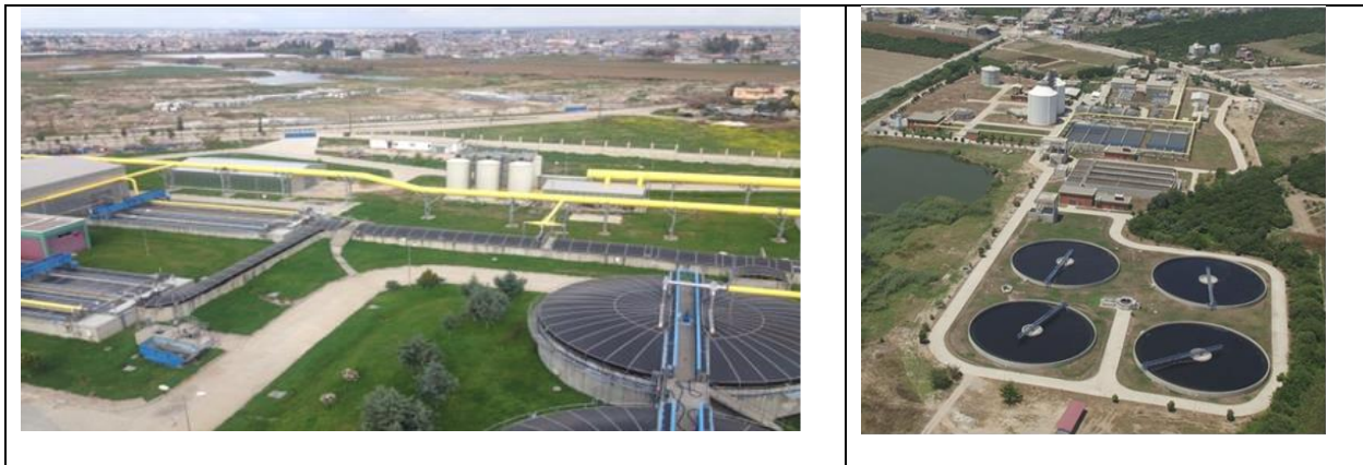
Figure 18. Yüreğir Wastewater Treatment Plant
