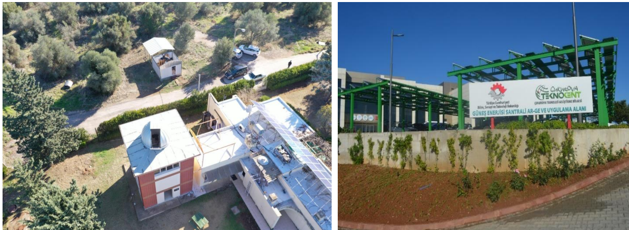
Figure 9 . PV Power Plant (Solar House and Technopark)
